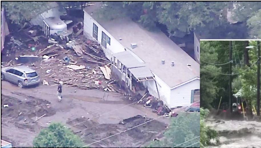
Homes damaged by flooding in Ruidoso. July 9, 2025. (KRQE Sky News 13)
